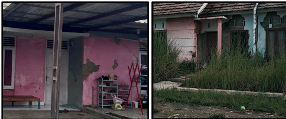
Figure 2. Occurrence of cracks and damage to the walls
